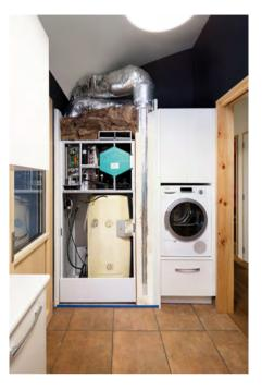
The 'magic box', housed in the laundry and coupled with a heat pump for hot water, provides heating, cooling and heat recovery ventilation and is a key part of the home's Passive House design.
